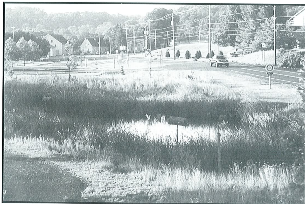
Wetlands function as filters and can be designed to treat runoff from roads and parking lots. (Photo: LandStudies, Inc.)
