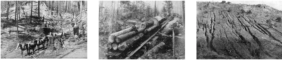
Figure 1-3. Early loggers worked their way through Pennsylvania and other states, denuding hillsides and causing massive erosion into stream and river valleys.
