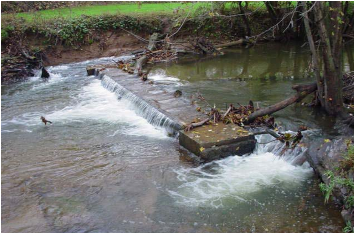
Figure 2-16. Former concrete pedestrian walkway at the Cove, now collapsed into the stream bed because of lateral migration of the channel, provides grade control.
