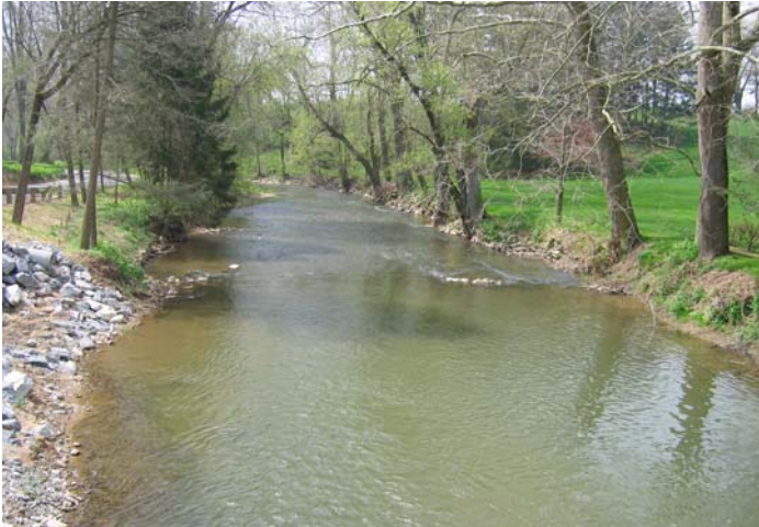
Figure 2-9. Looking downstream from below the Longenecker Road bridge crossing. Longenecker Road can be seen immediately adjacent to the stream channel on the far left. Note riprap material on the left bank as an attempt to minimize bank erosion. Also note along the right bank the leaning trees, which will eventually fall and create debris jams.
