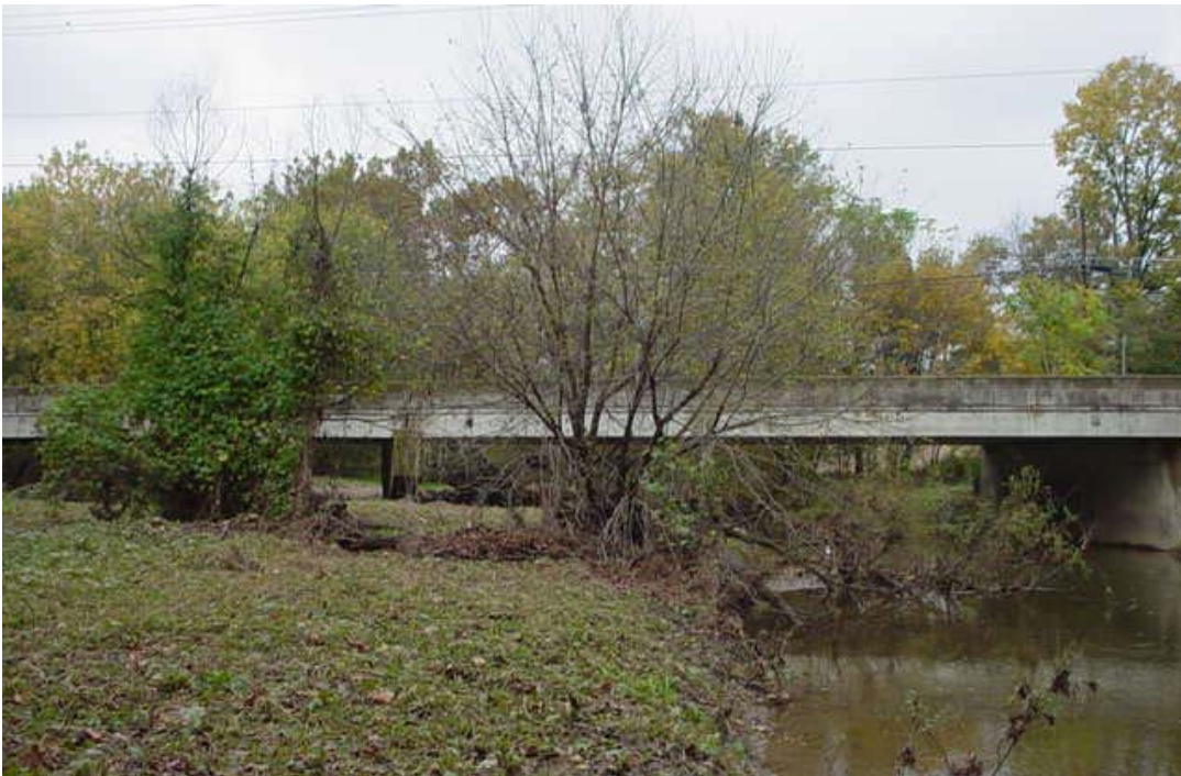
Figure 2-15. Route 772 Bridge Crossing, looking upstream.
