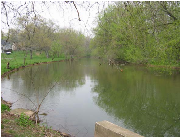
Figure 2-12. Looking upstream from Sico Dam, the ponded backwater behind the dam is obvious.
