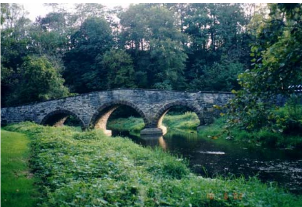
Figure 2-6. A proper alignment between channel and bridge opening would show the stream flowing toward the bridge from the lower left-hand corner of the photograph. The acute angle of approach in the existing condition suggests that the channel may have migrated from its original path.
