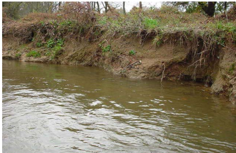
Figure 2-28. Sections of Brubaker Run are deeply incised with high, eroding banks, similar to conditions found through the Little Chiques main stem.
