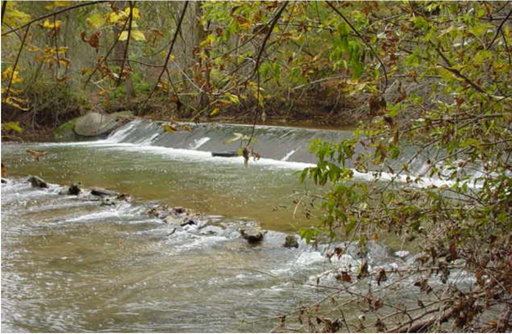
Figure 2-17. Deteriorating dam at the upper end of the Cove area.
