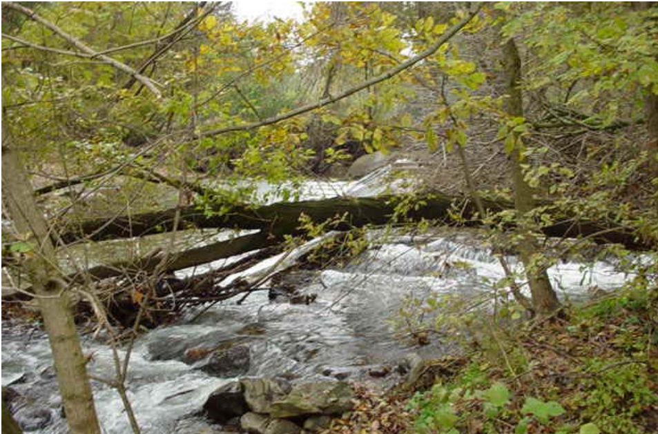
Figure 2-18. The Little Chiques Creek channel has breached the dam, shown here along the left bank. Debris jams created by fallen trees are common occurrences throughout Little Chiques Creek and indicate a substantial amount of lateral erosion and stream bank undercutting.
