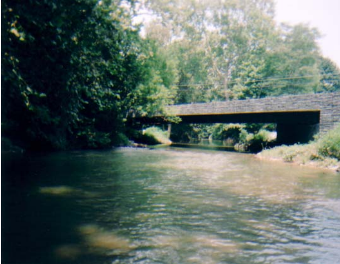
Figure 2-10. Looking upstream to the Longenecker Road bridge crossing.
