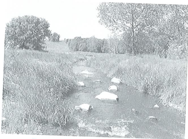
Octoraro Nursery stream restoration project
